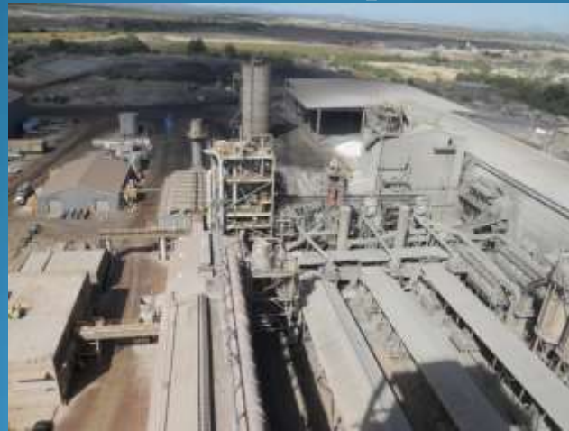
Rillito Cement plant
